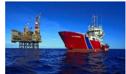
Laser controls boat position to oil rig
